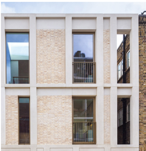
Concrete and inset brickwork
