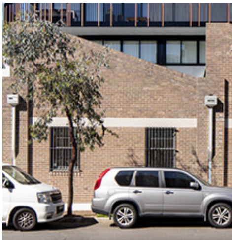
Splayed brick parapet
