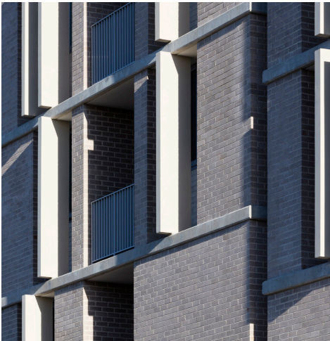
Expressed concrete slabs
