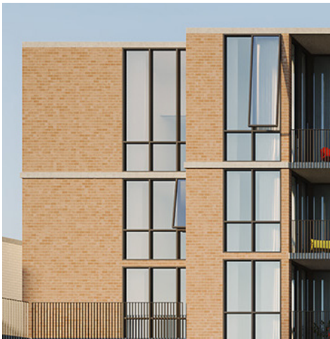
Full height strip windows
